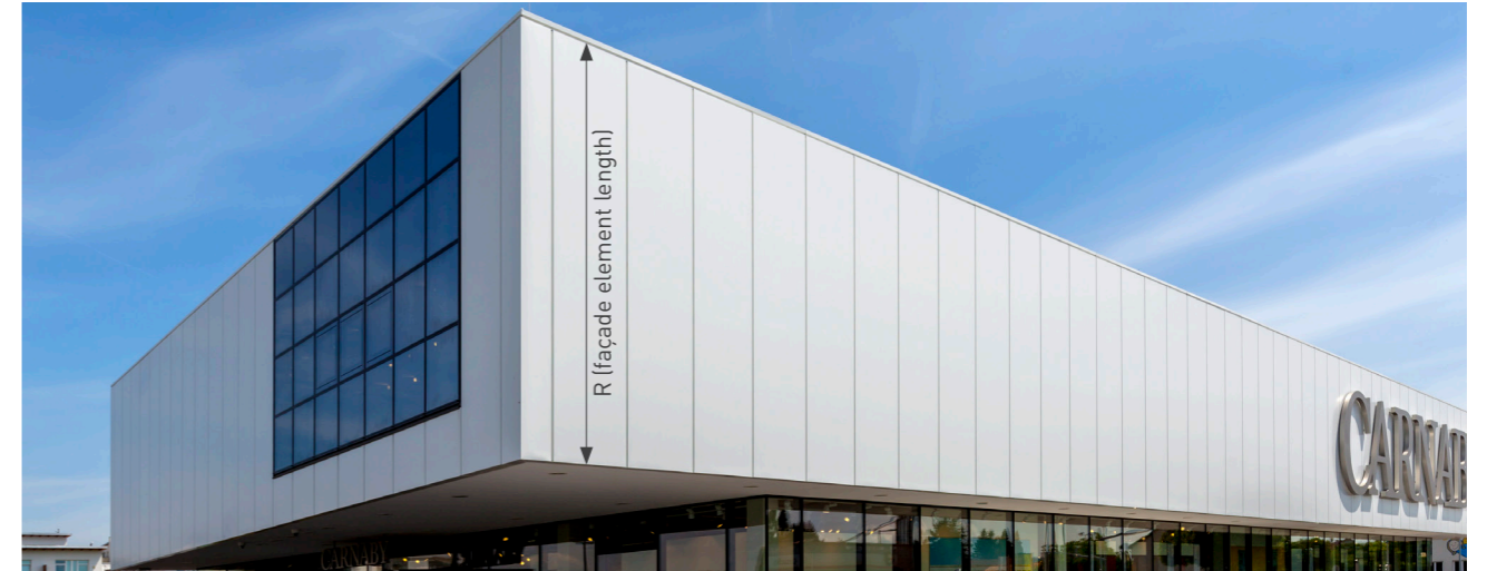
Qbiss Screen longitudinal corner element completing building envelope.
